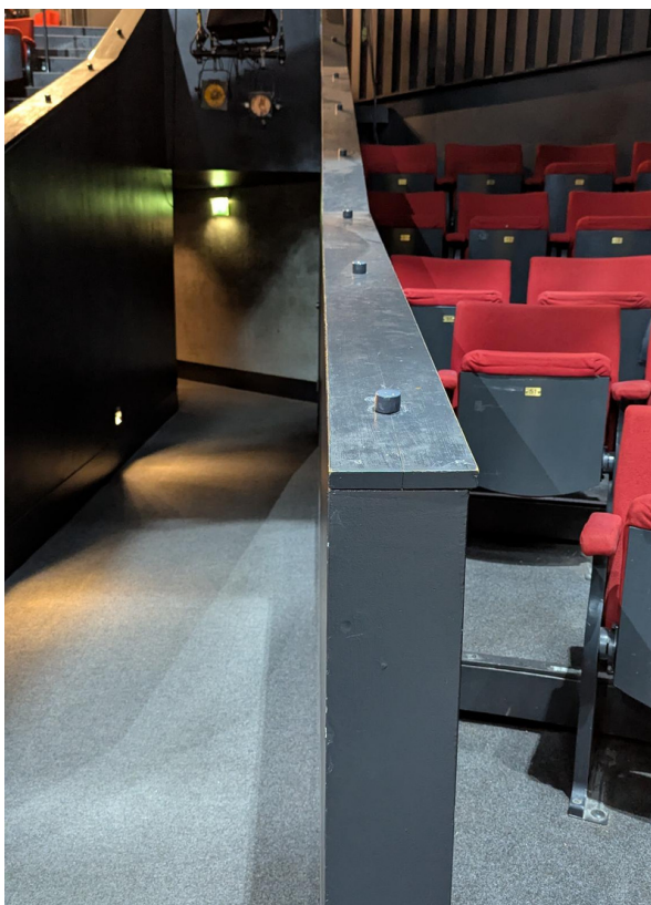
Wall next to seats #51 (no aisle access)
